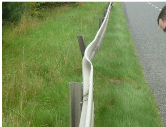
Figure 5.3 - Medium & Low Priority Damage: No design required
