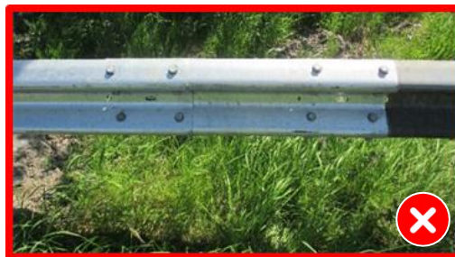
Figure 3.20 - Short cut pieces are not permitted
