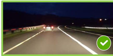
Figure 2.11 - Example of VRS reflector colours on a single carriageway: red on nearside, white on offside
