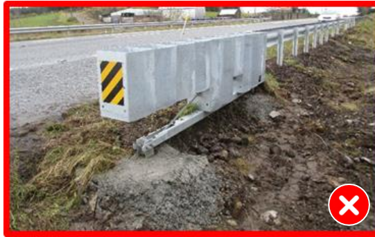
Figure 5.13 - Verge re-profiling works required at replacement terminal
