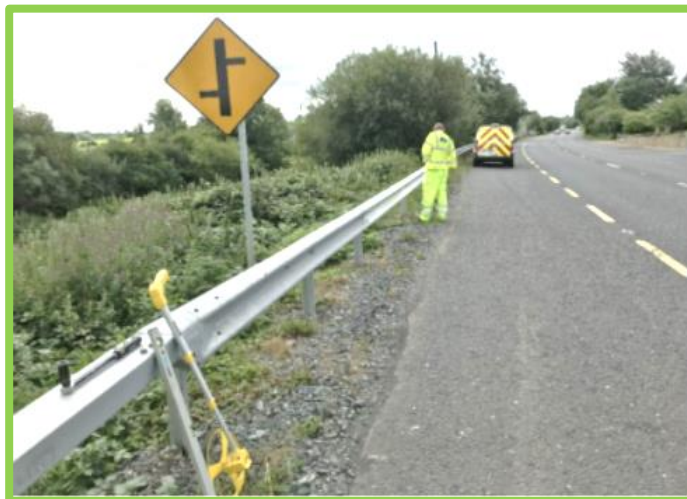
Figure 4.11 - VRS inspection underway
