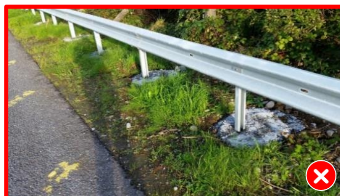
Figure 3.31 - Example of exposed concrete foundations
