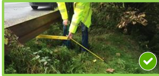
Figure 4.21 - Verge profiling being checked during detailed inspection of an existing VRS
