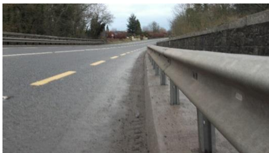
Figure 5.5 - Full Replacement Barrier: Design input required
