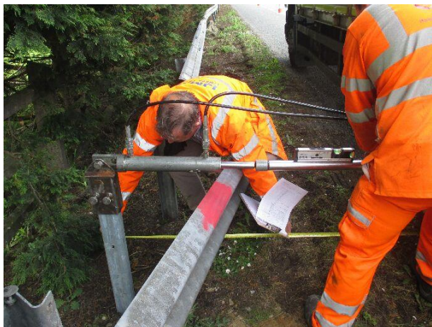
Figure 3.32 - Push testing in progress
