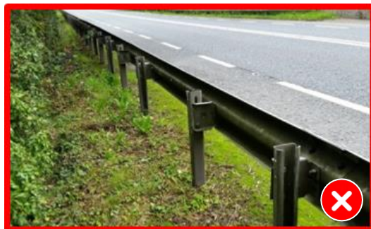
Figure 4.18 - Example of posts orientated in opposite directions
