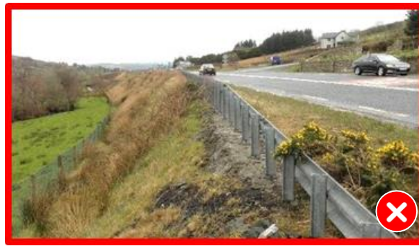
Figure 3.22 - Example of constrained location with minimal/no working width available
