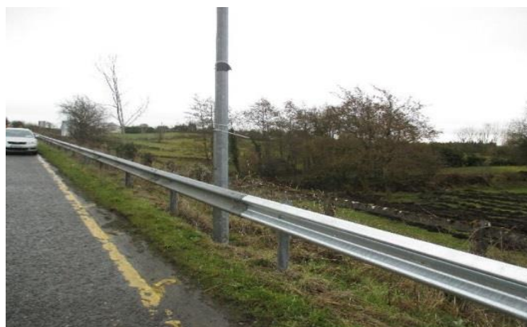
Figure 4.14 - Lighting column within barrier working width
