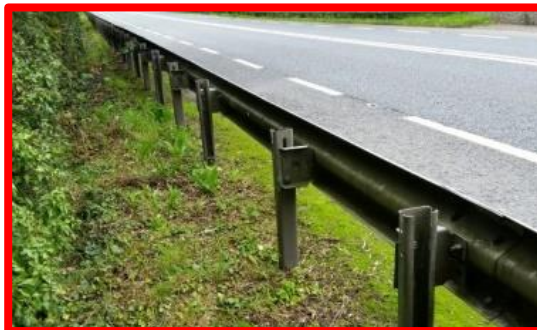
Figure 5.8 - Example of posts orientated in opposite directions
