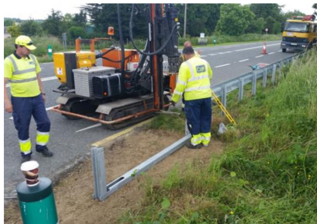
Figure 3.12 - VRS repair works underway
