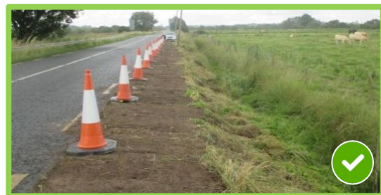
Figure 5.14 - Verge re-profiling works carried out prior to VRS installation
