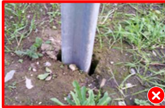
Figure 3.23 - Example of driven post moving in the ground
