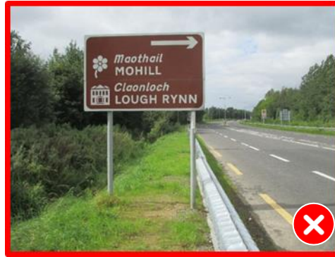
Figure 2.13 - Sign support within working width of terminal
