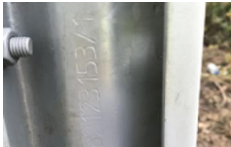
Figure 2.16 - Example of Traceability Marking on VRS post
