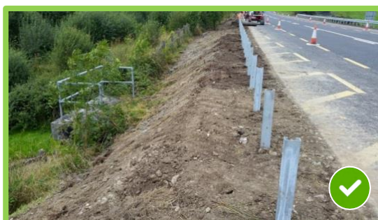
Figure 5.15 - Example of verge re-shaped and reinstated with existing topsoil
