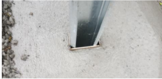
Figure 5.9 - Example of post in socket
