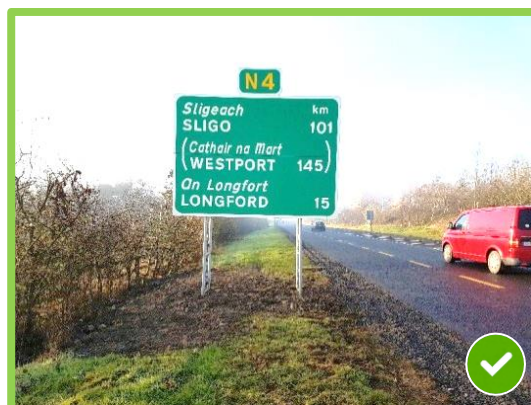
Figure 5.1 - Sign installed on passively safe posts to enable complete removal of a damaged VRS
