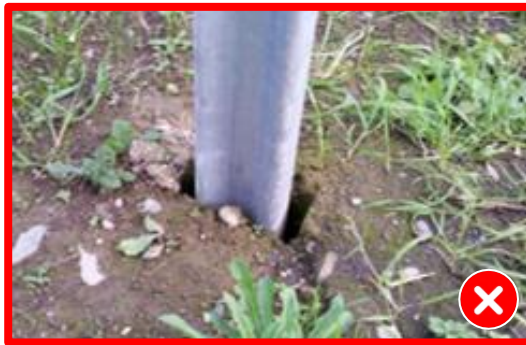
Figure 4.17 - Example of driven post moving in the ground
