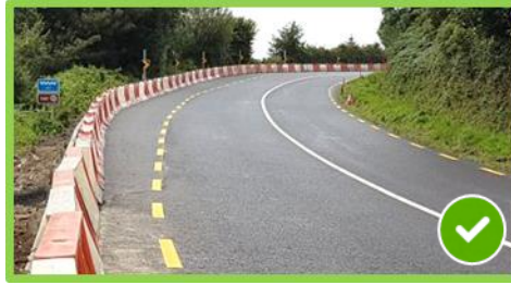
Figure 3.4 - Example of damaged VRS protected by temporary barrier
