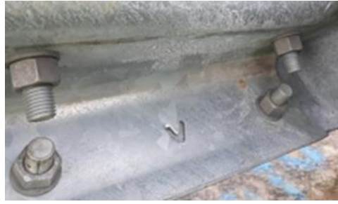
Figure 2.15 - Example of Traceability Marking on VRS beam ('v' stands for Volkmann & Rossbach, Germany)
