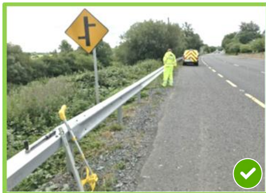
Figure 3.14 - VRS snagging underway
