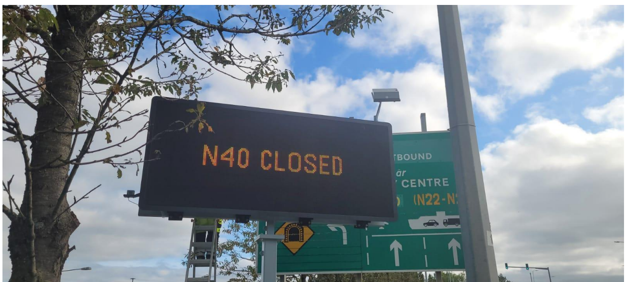
Photograph 4.3 Example of an Urban VMS (Post-Mounted)
