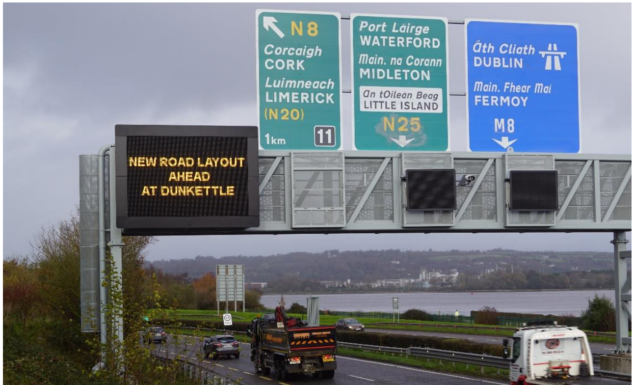
Photograph 4.2 Example of a Tactical VMS (Portal gantry-Mounted)
