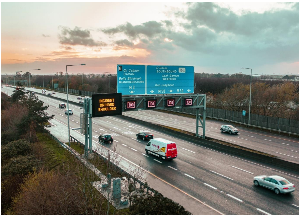
Figure 3.6 Lane Control Signs
