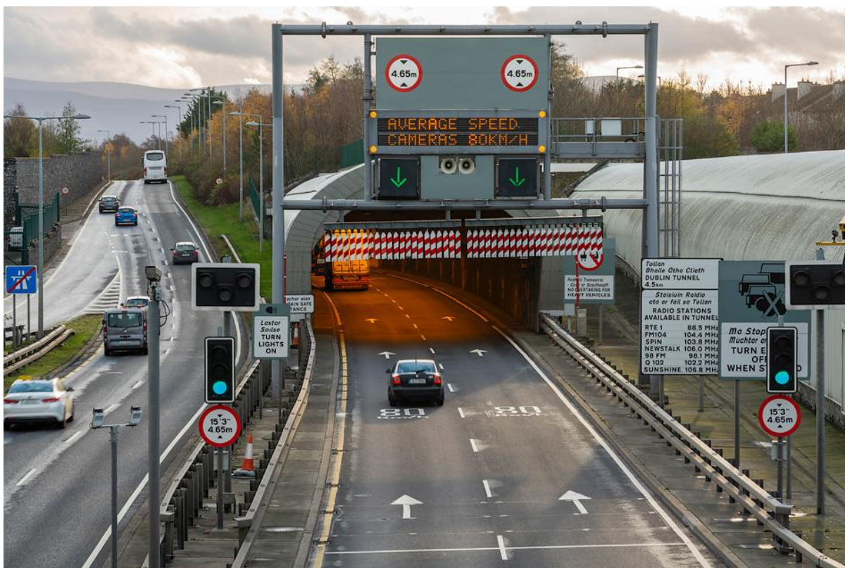
Figure 2.1 Variable Message Sign at Dublin Tunnel
