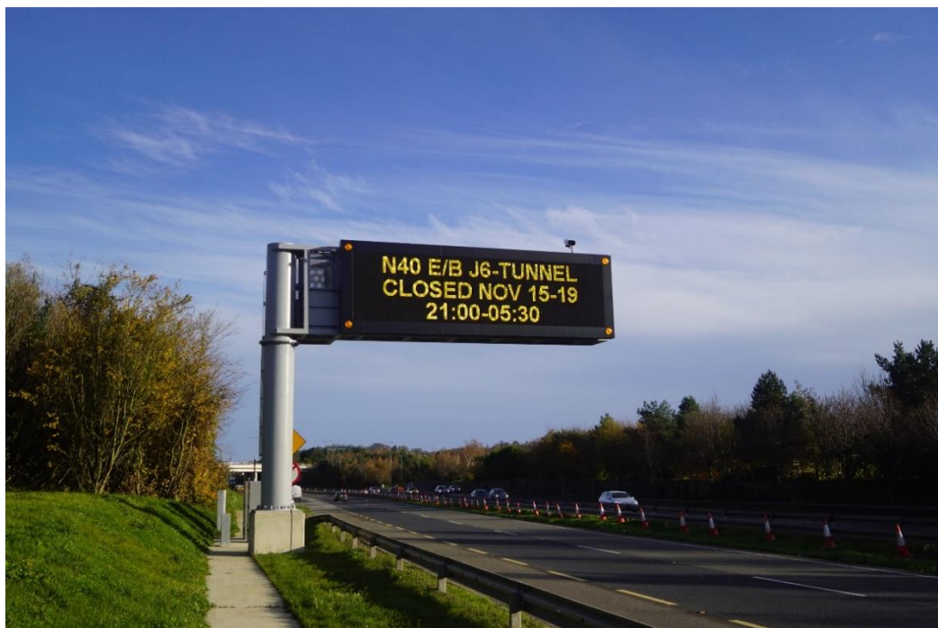
Figure 3.2 Existing cantilevered VMS
