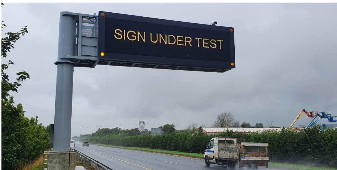
Figure 5.1 Test message on VMS
