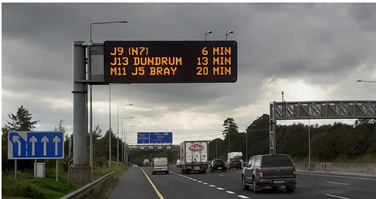
Figure 3.5 Single Colour Full Matrix VMS
