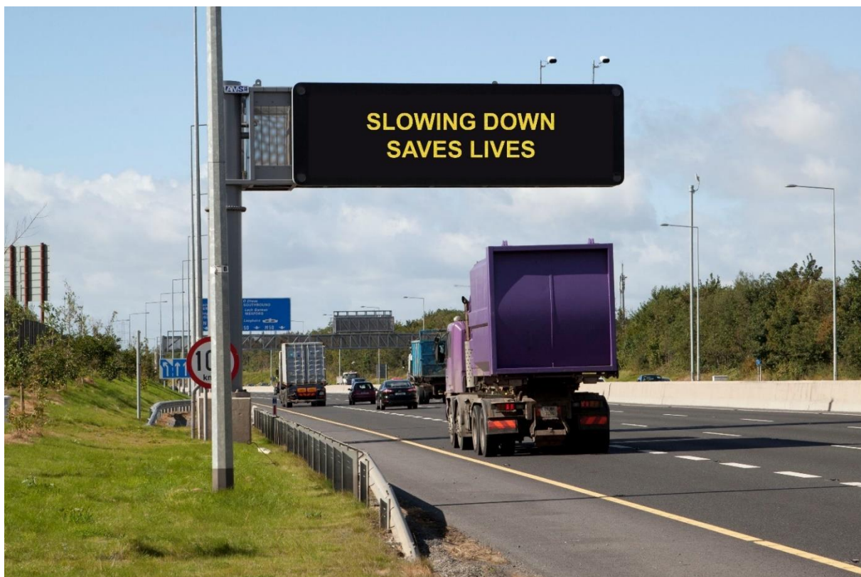
Figure 4.2 VMS Displaying Safety Message
