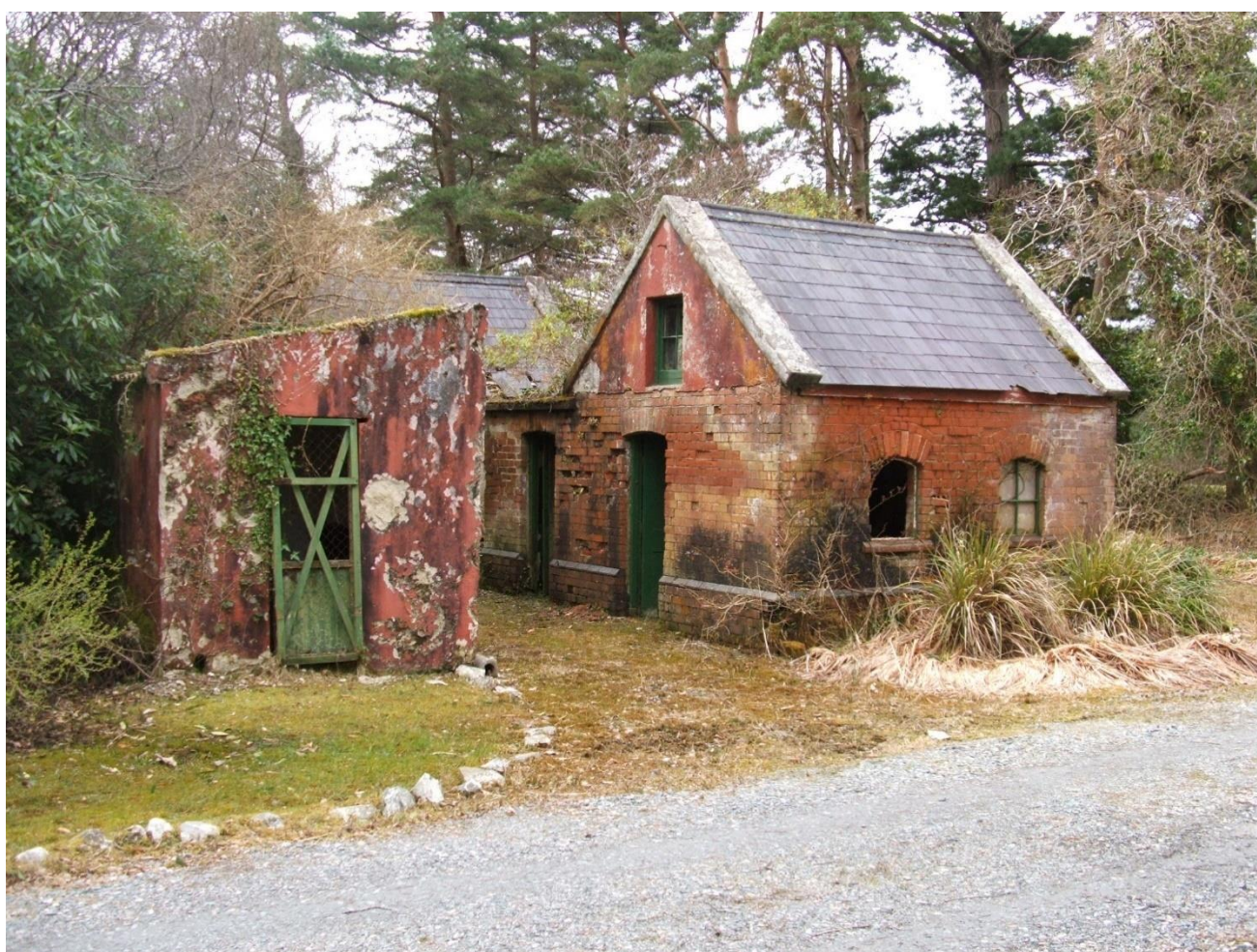
Illustration 5—There is a rich legacy of Victorian railway buildings along the old Galway to Clifden line (1895–1935). Galway County Council is bringing the disused railway line back to life after almost 100 years as the route of the Conamara Greenway project. (Photo: TII Archaeology and Heritage)
