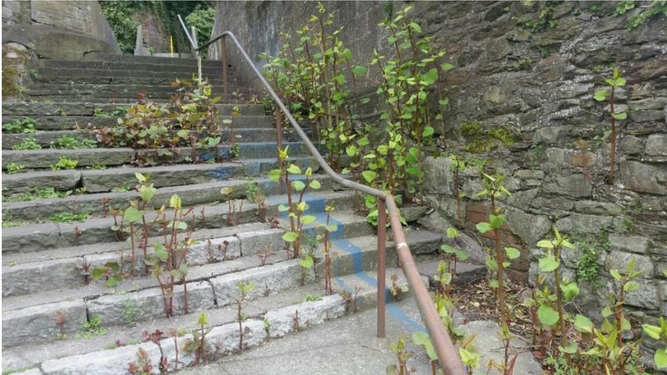
Figure 1 Japanese knotweed breaking through a paved surface [Photo: Arup]
