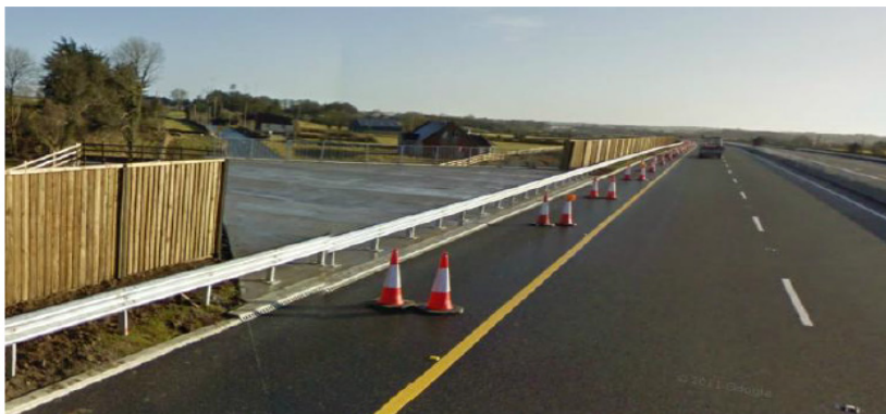
Figure B.9 - Break in barrier continuity at bridge section
