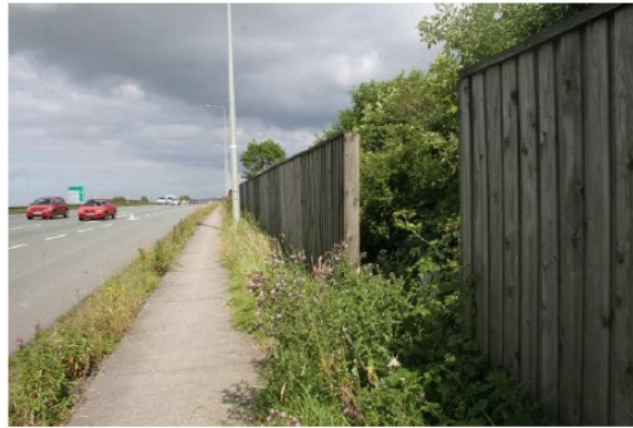
Figure B.9 - Break in barrier continuity at bridge section
