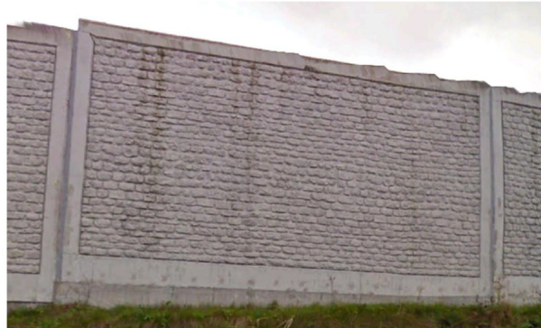
Figure B.16 - Concrete Barrier
